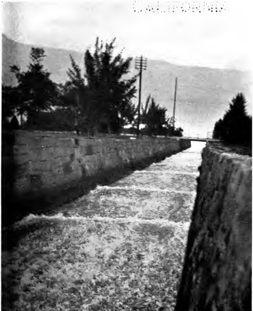
ROLL-WAVES IN THE GRÜNNBACH CONDUIT, LOOKING DOWN-STREAM.
